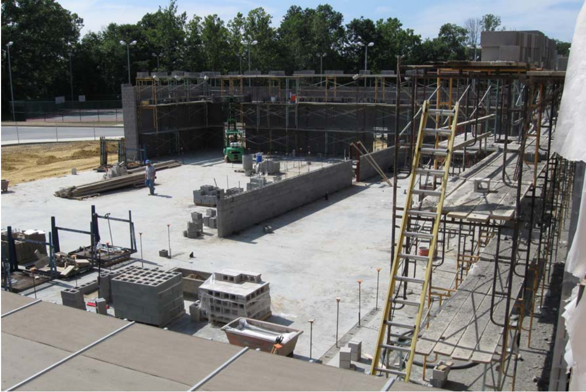
Band/Orchestra Addition – Exterior Walls Being Installed
