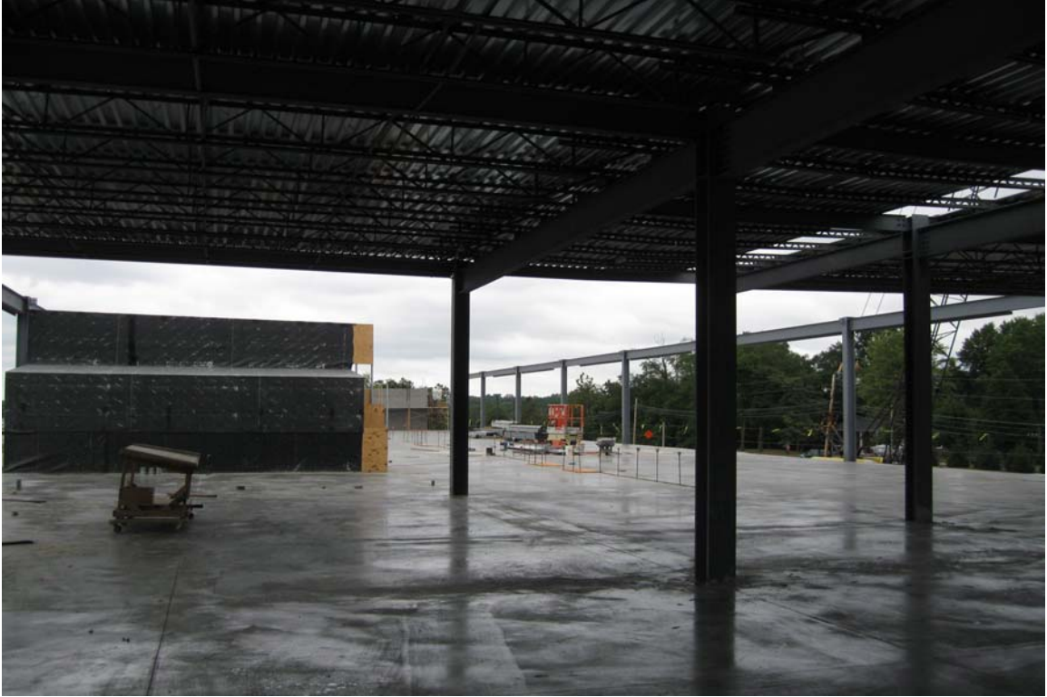
Two Story Addition – 2 nd Floor (Looking West)
