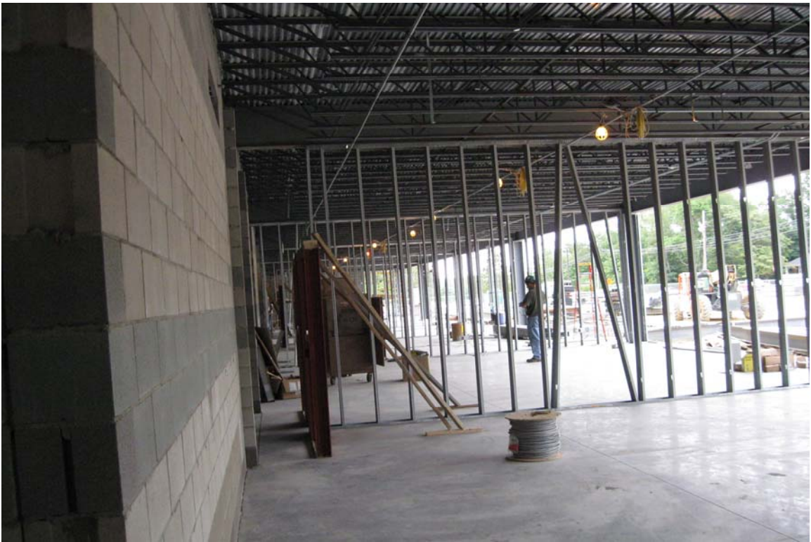
Two-Story Addition – 1 st Floor (Looking West)
