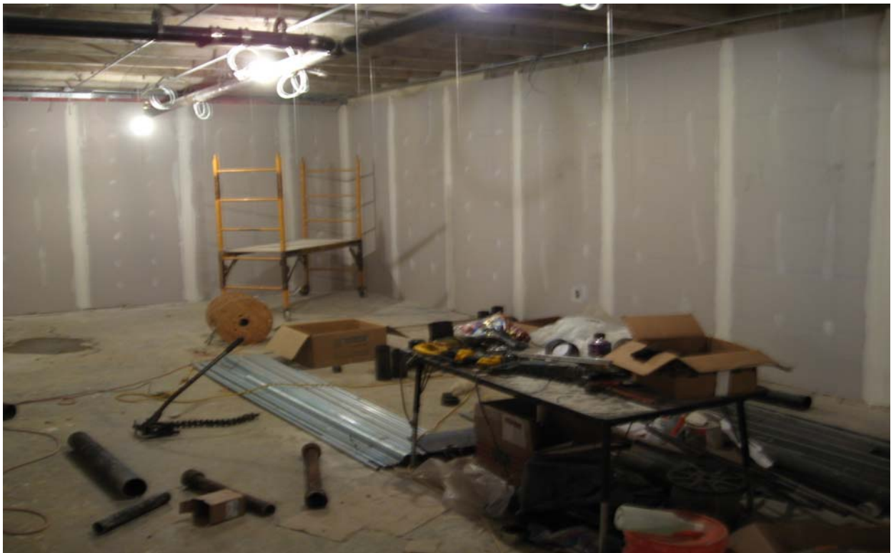
Electrical & Mechanical Rough-Ins and Drywall Installation at the New ROTC area
