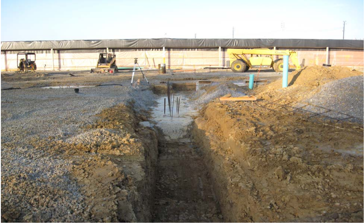
Exterior Foundation Work at the New 2-Story Addition
