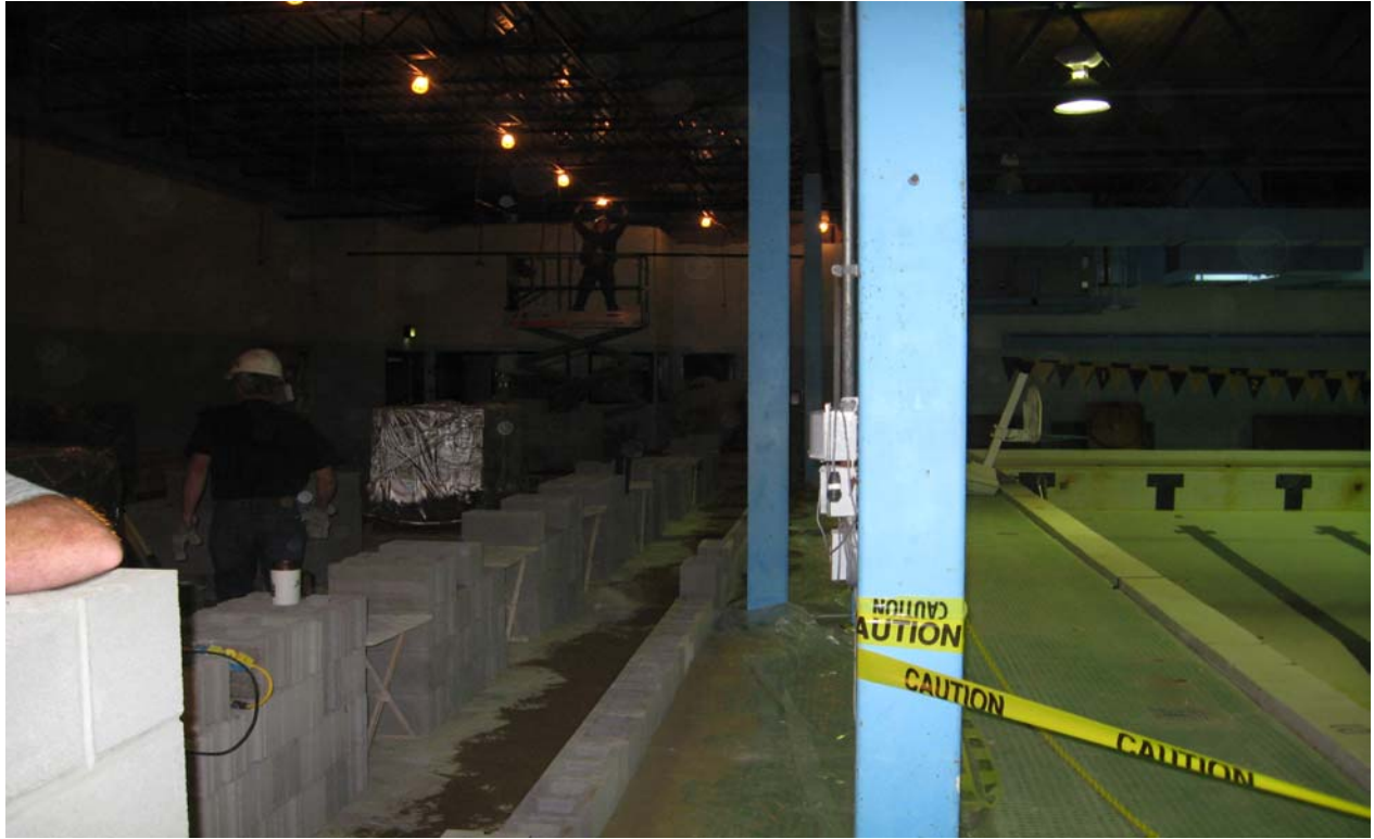
Masonry Wall installation in Pool Area
