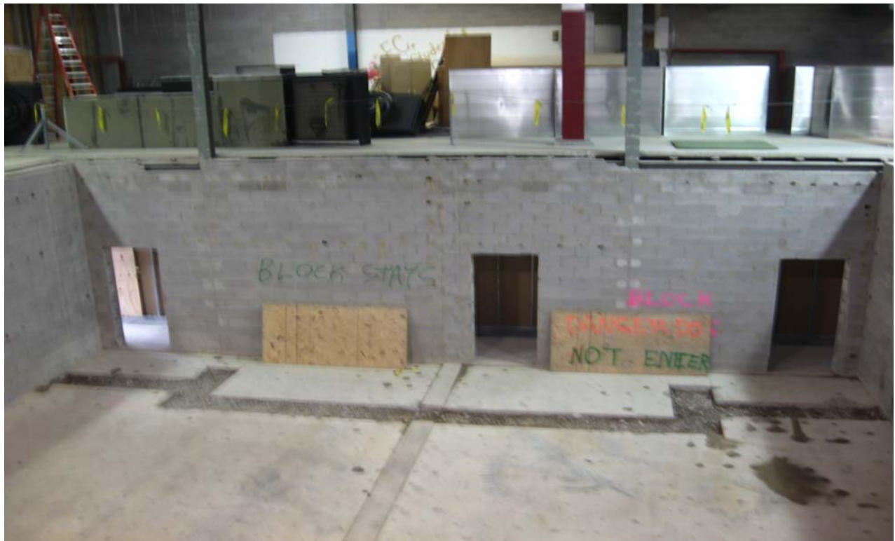
Demolition of the Old Racquetball Courts
