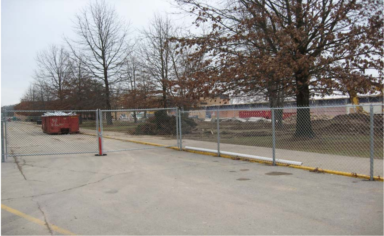
Temporary Fencing at New 2-Story Addition Area
