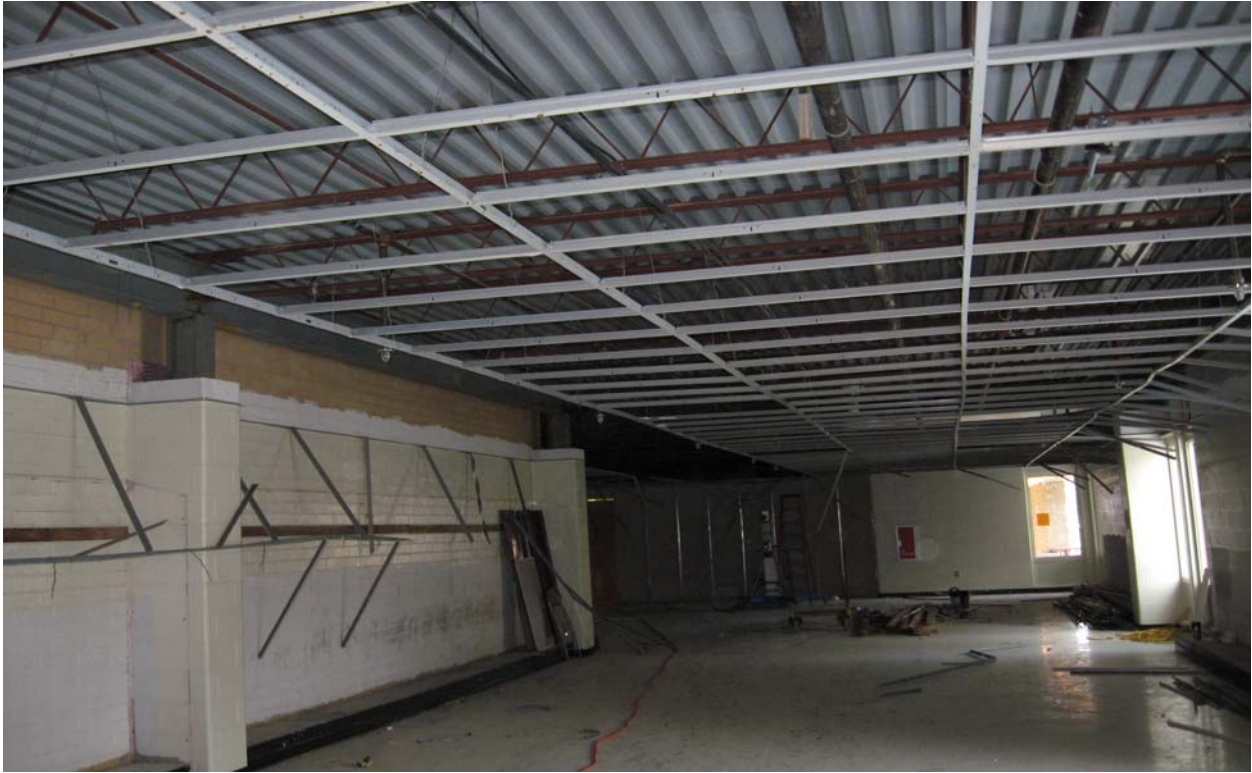
Interior Demolition nearly Complete at New Art Rooms Addition
