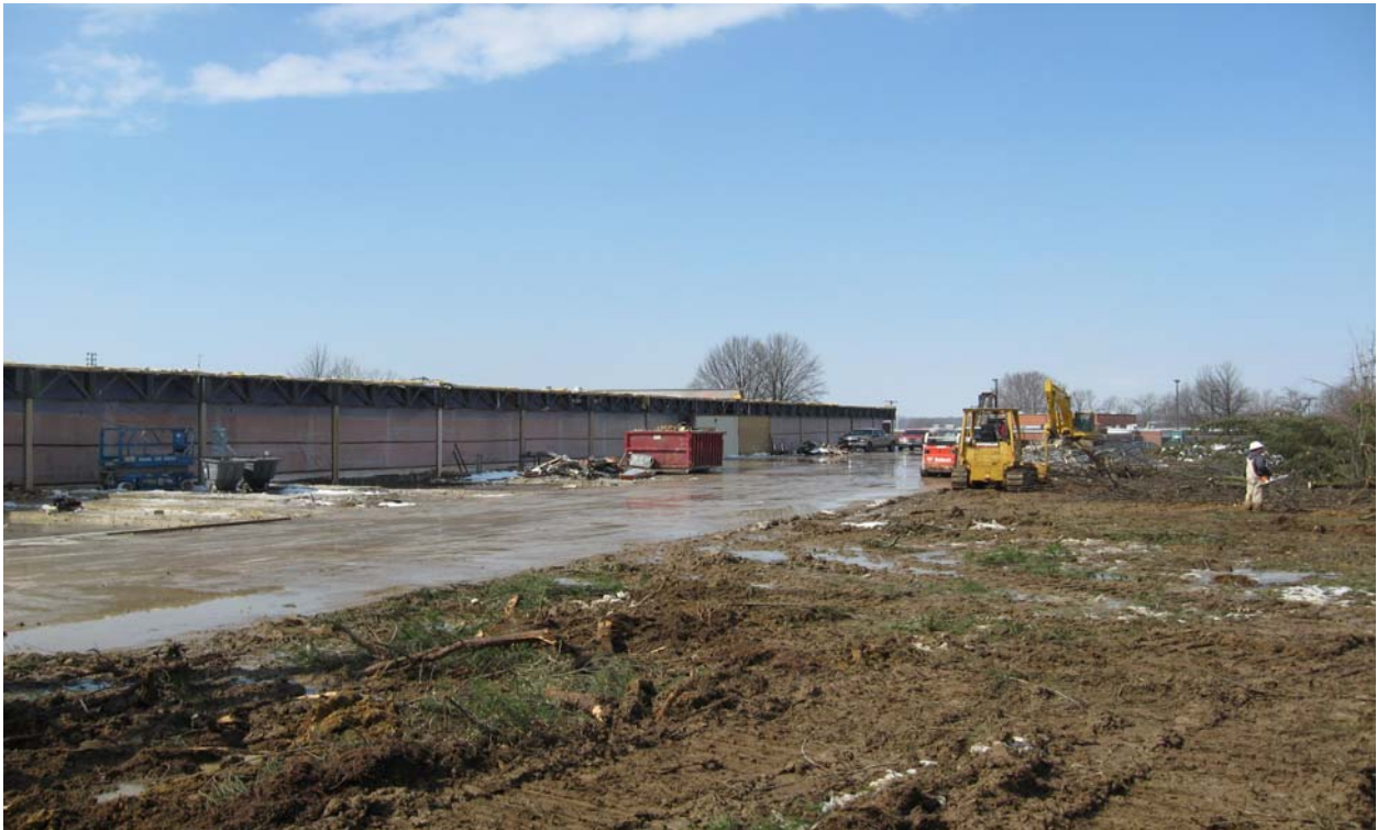
Existing Structure Removed at New 2-Story Addition Area
