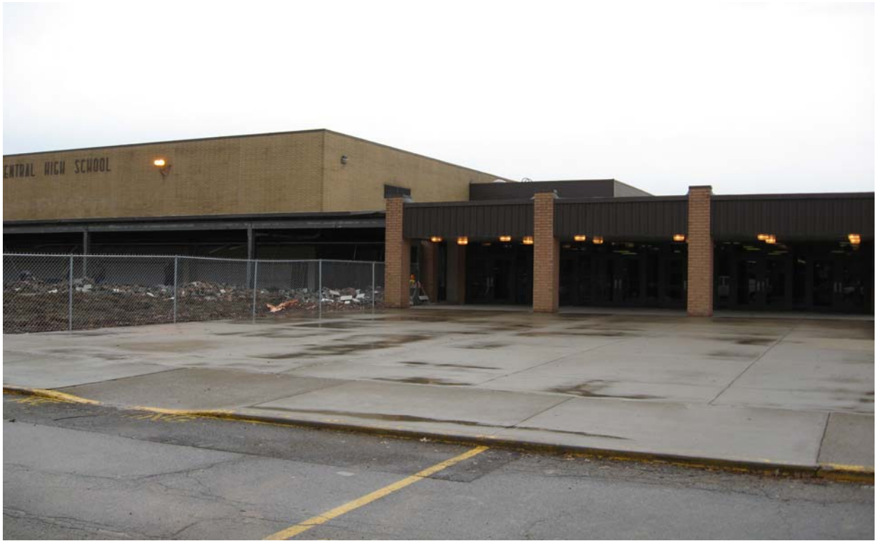
Existing Structure to be Removed at the New Art Room Addition
