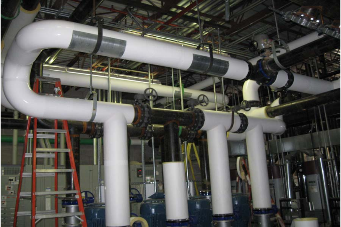
Mechanical Room Work
