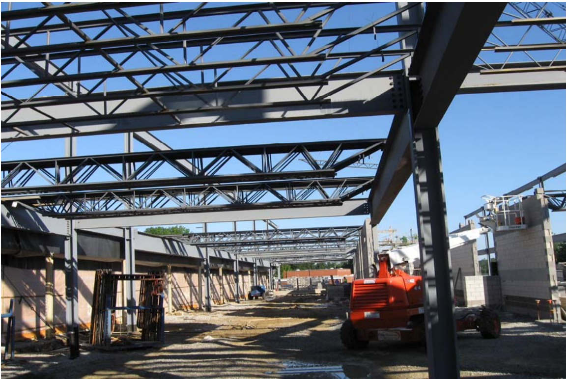
2 nd Floor Joist at New Classroom Addition
