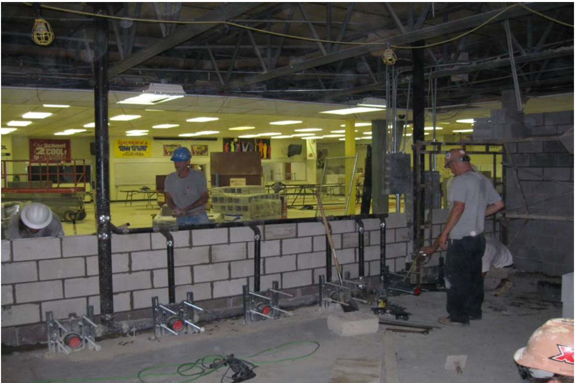
New Restrooms near Kitchen and Cafeteria
