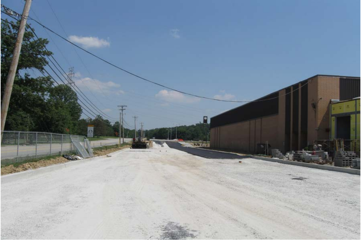
Asphalt Paving at Front of School
