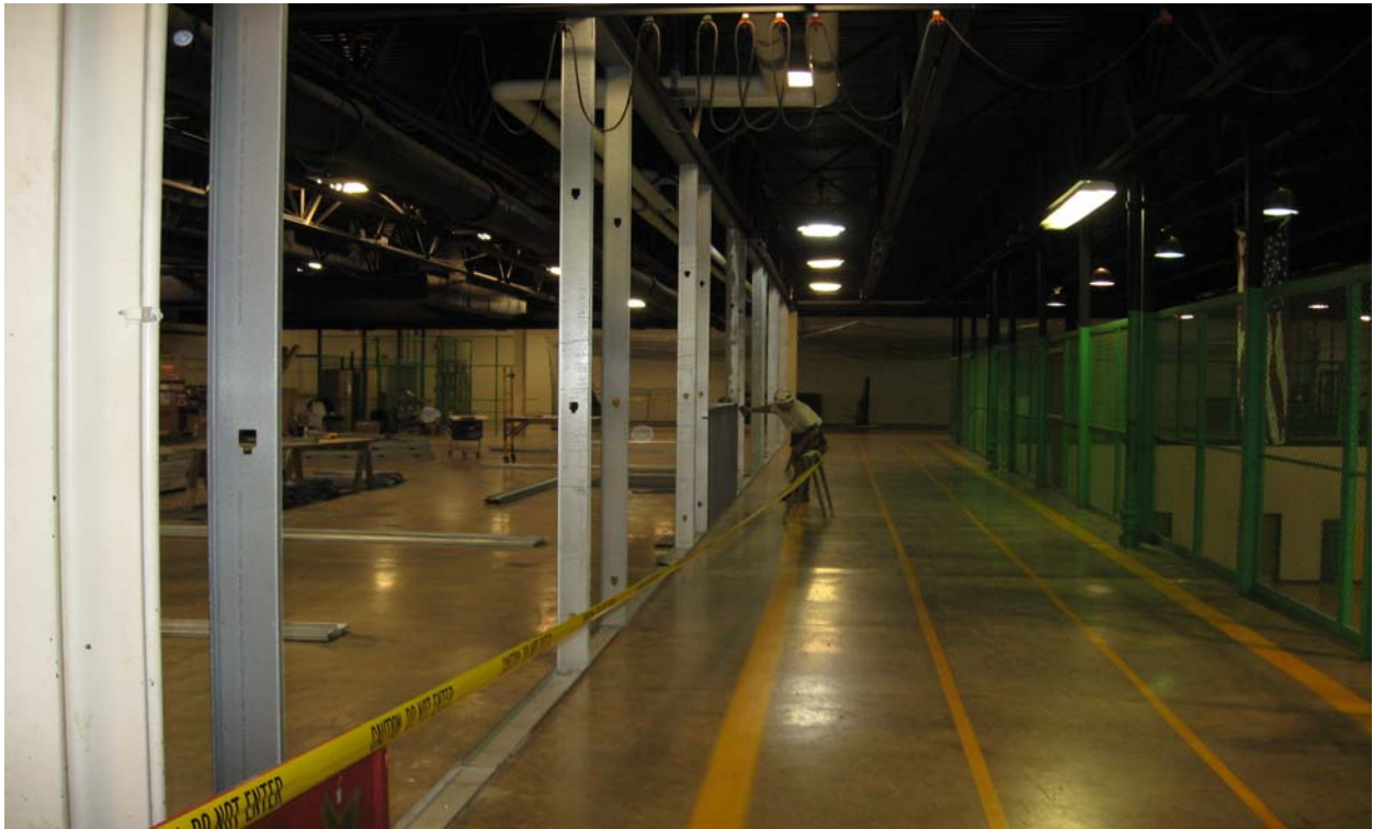
Framing of New Wrestling Area on 2 nd Floor of Unit "C"
