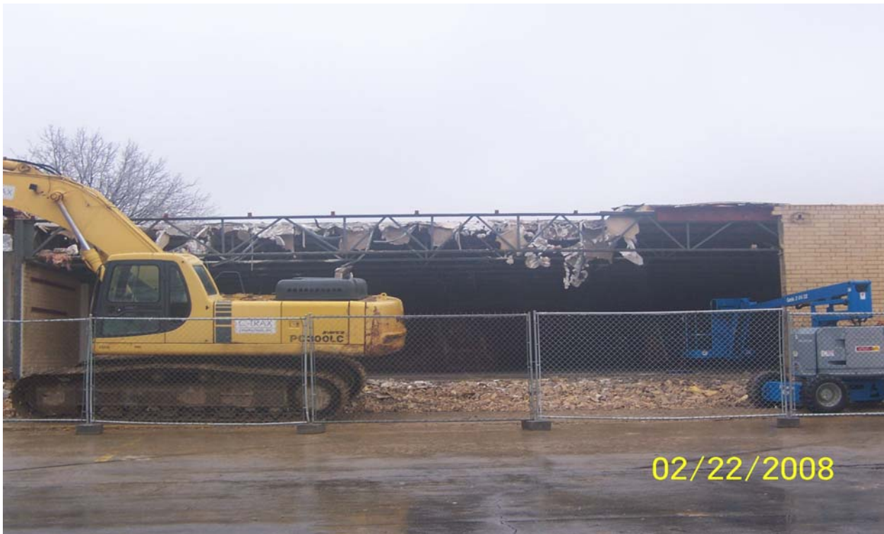
Demolition of the Existing Building has Started
