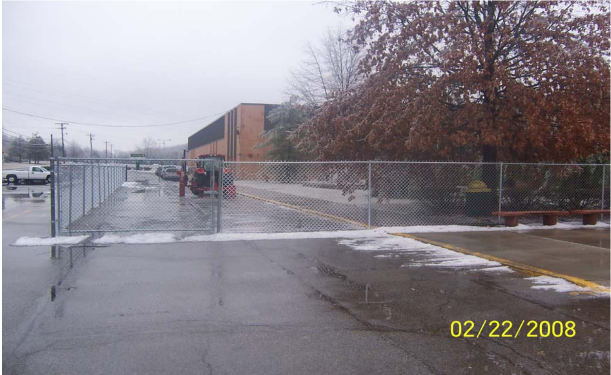
Temporary Fencing at the Front of the School
