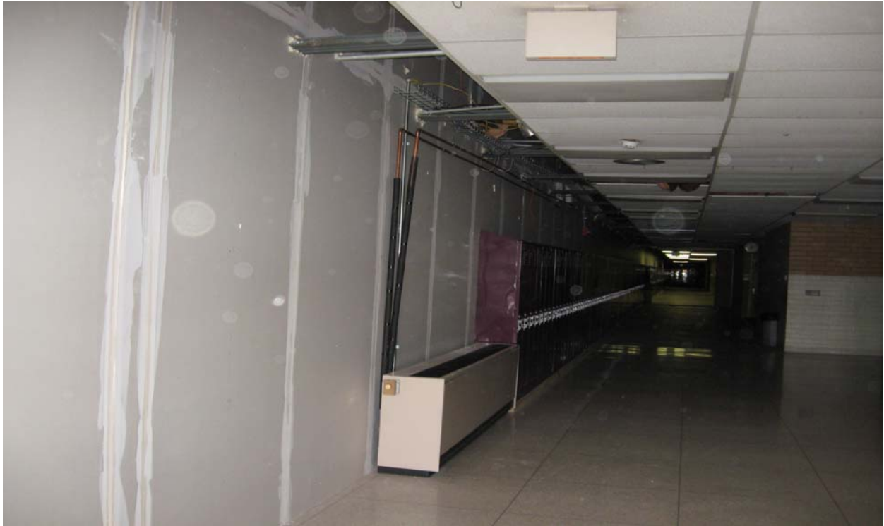
Temporary Wall for Structural Removal to Start
