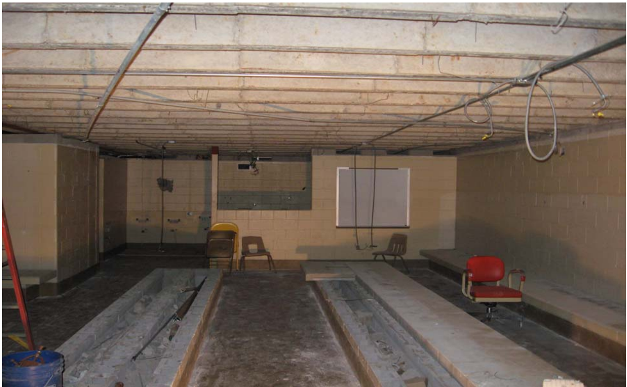
Demolition of Main Gym Locker Rooms
