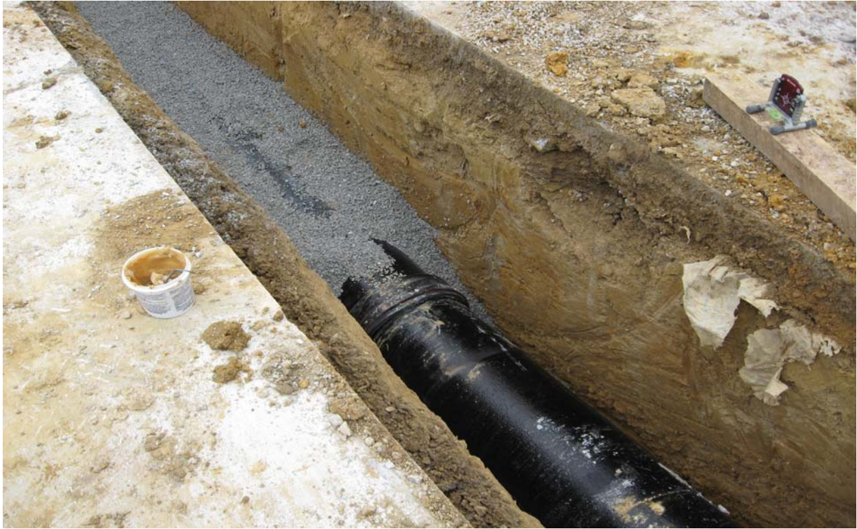
Underground Storm Sewer at New 2-Story Addition Area
