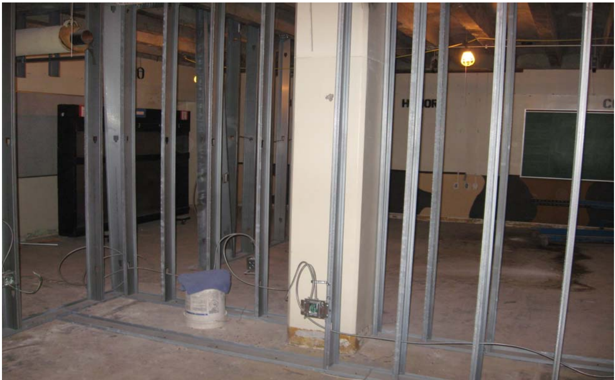
Metal Stud Walls and Electrical Rough-Ins at the New ROTC area
