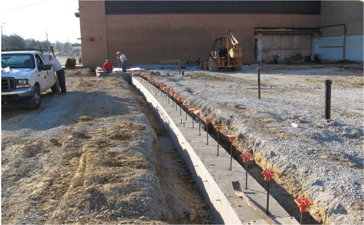
Exterior Foundation Wall at the New Art Rooms Addition
