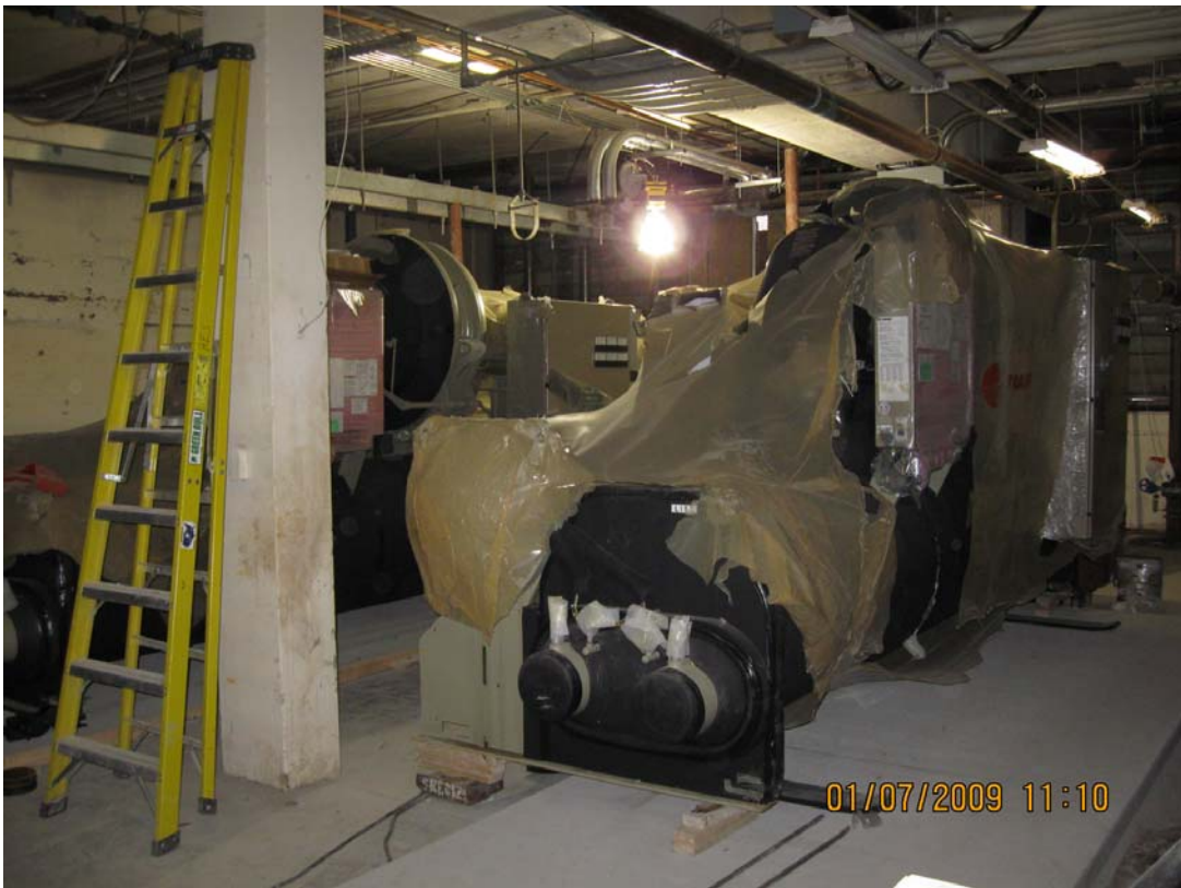
Setting of New Chillers
