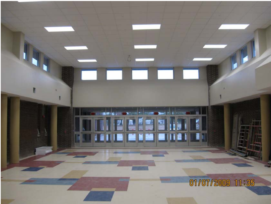
New Entrance at Bus Parking Lot
