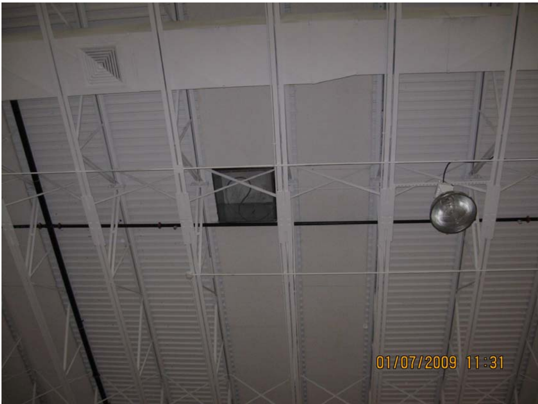
Erection of Acoustical Panels at Auxiliary Gym
