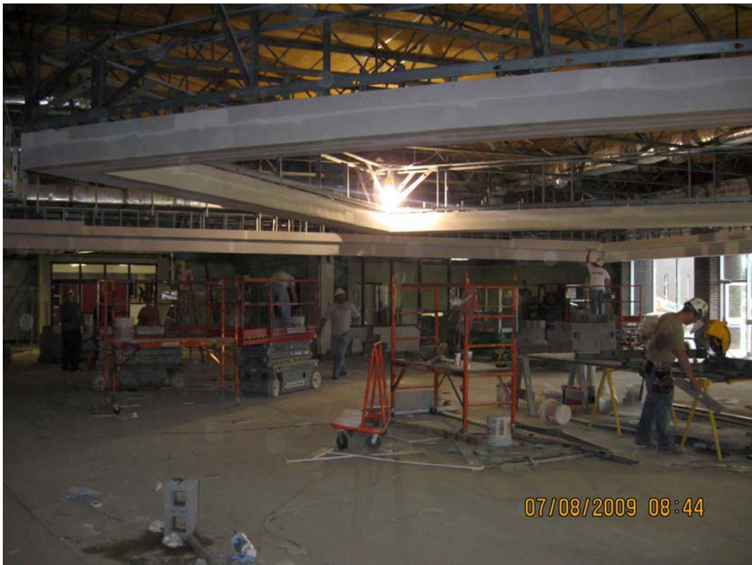
Erection of Bulkhead within Media Center
