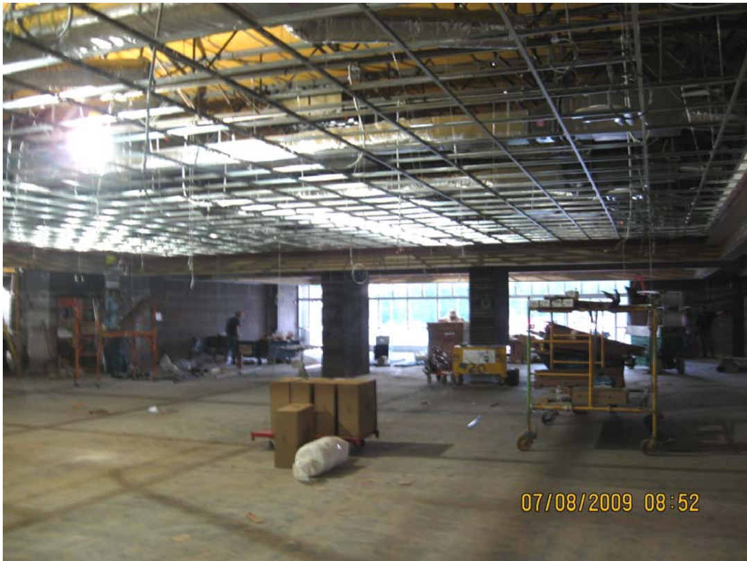
Installation of Ceilings within Cafeteria
