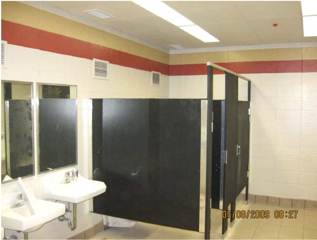
Renovated Restrooms on 2 nd Floor
