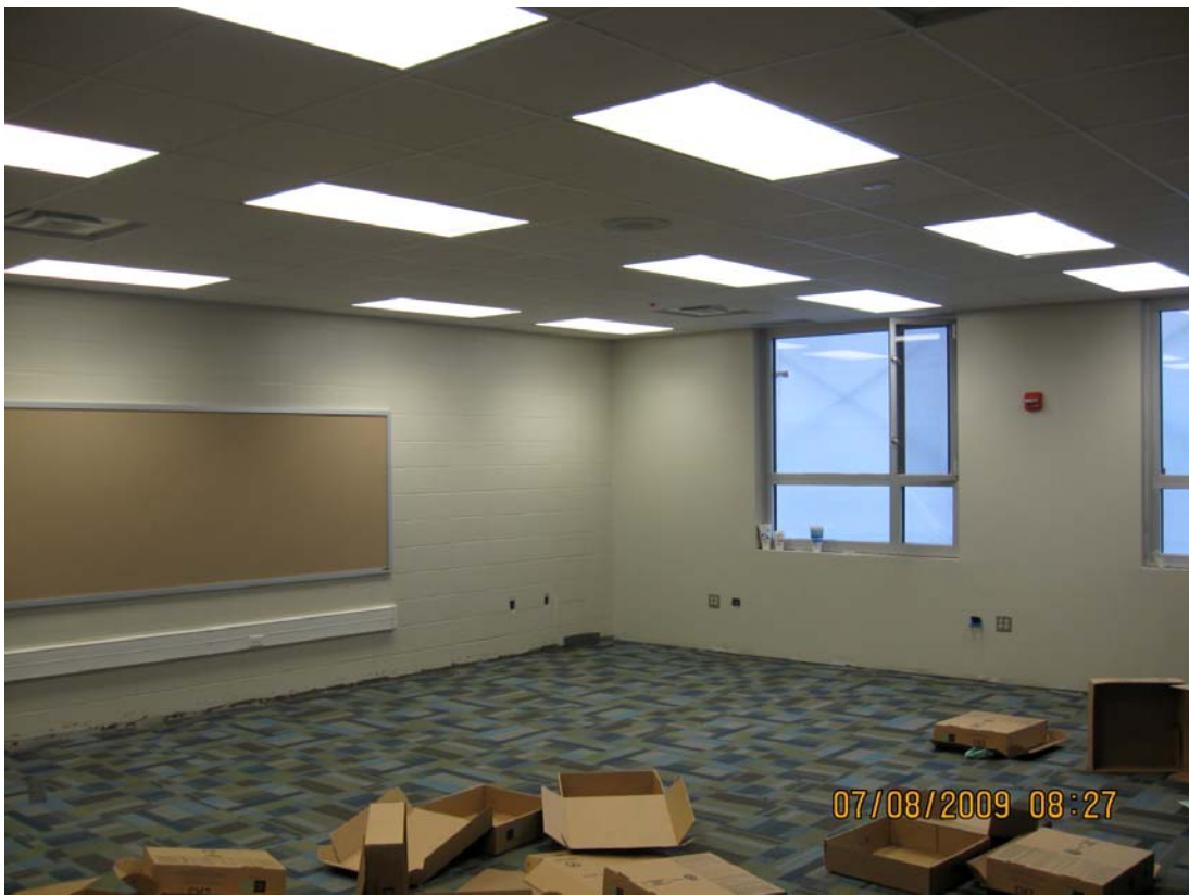
Renovation of 2 nd Floor Classrooms
