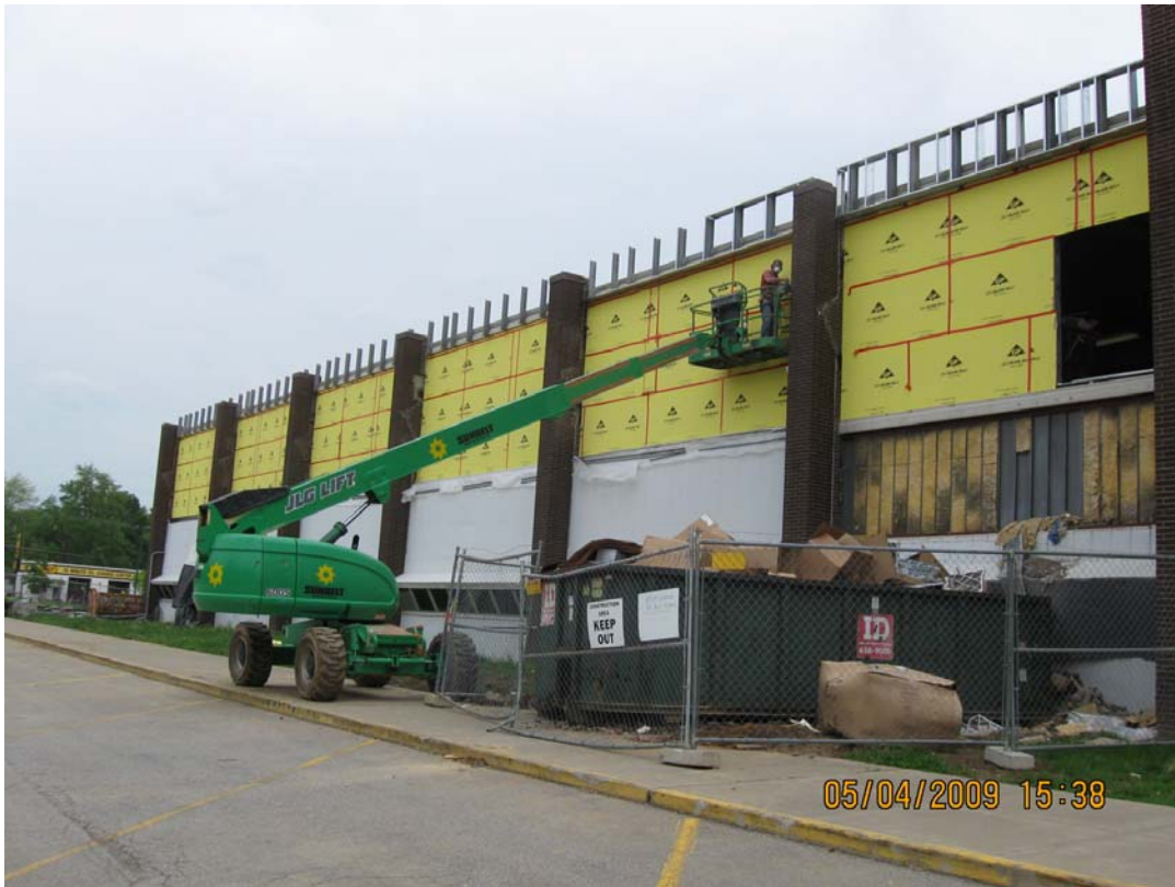
Re-skinning of the North Elevation
