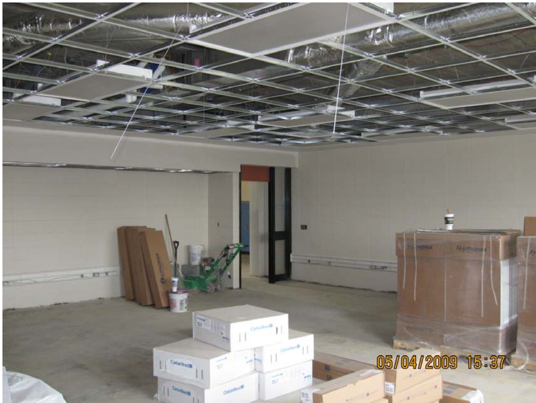
Renovation of the Remaining Classrooms on the 2 nd floor
