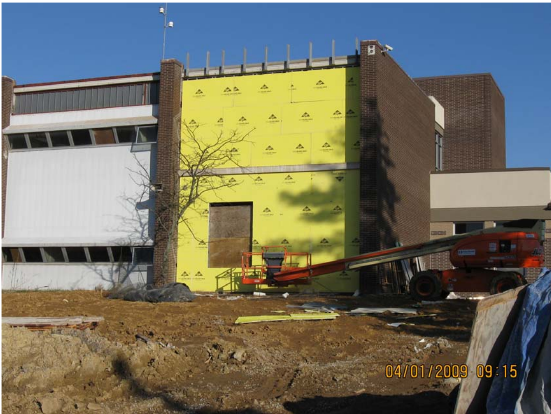
Erection of new building skin along South elevation
