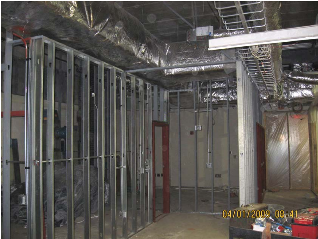
Erection of new walls @ Old Administration Area
