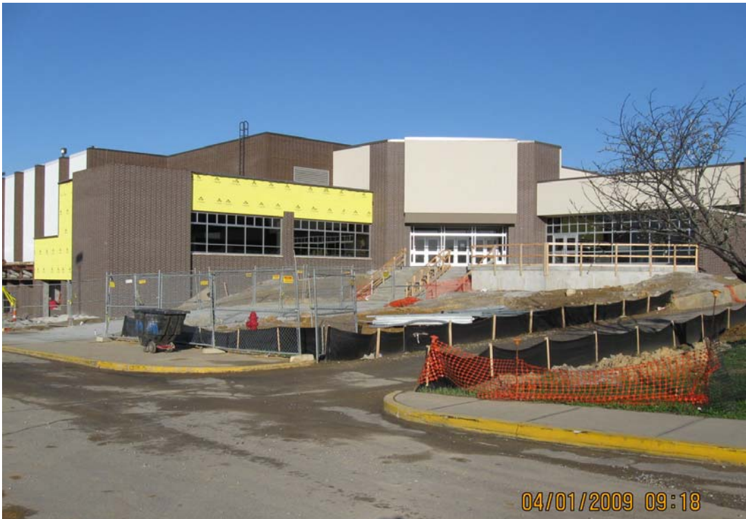
Enclosure of Units F and J
