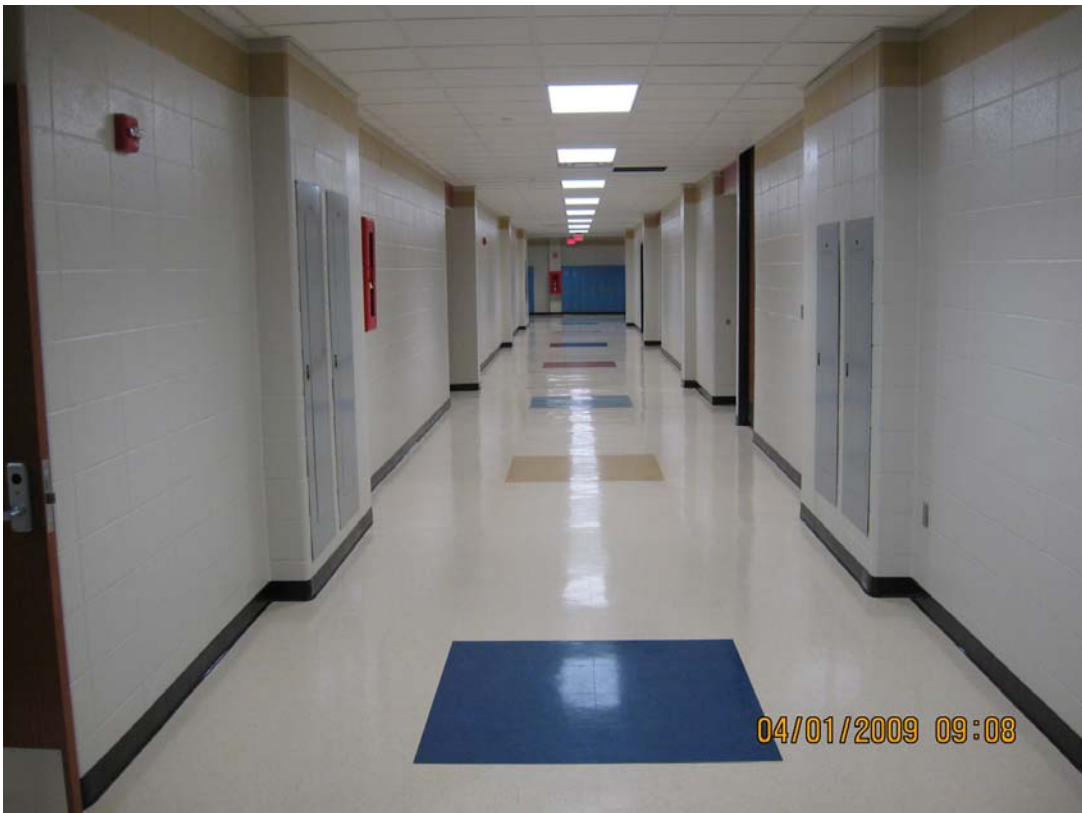
Interior finishes @ 2 nd floor, middle corridor
