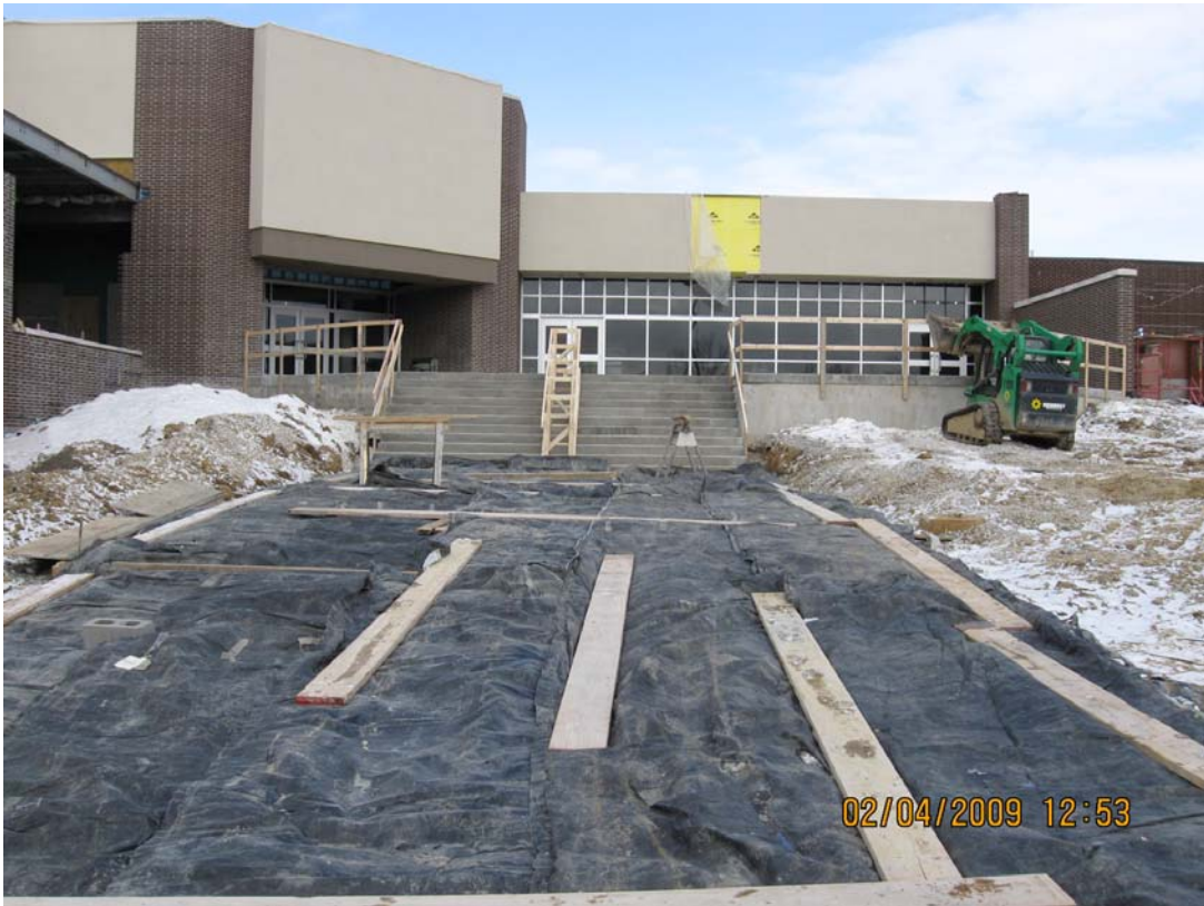
Placement of Cafeteria patio and steps
