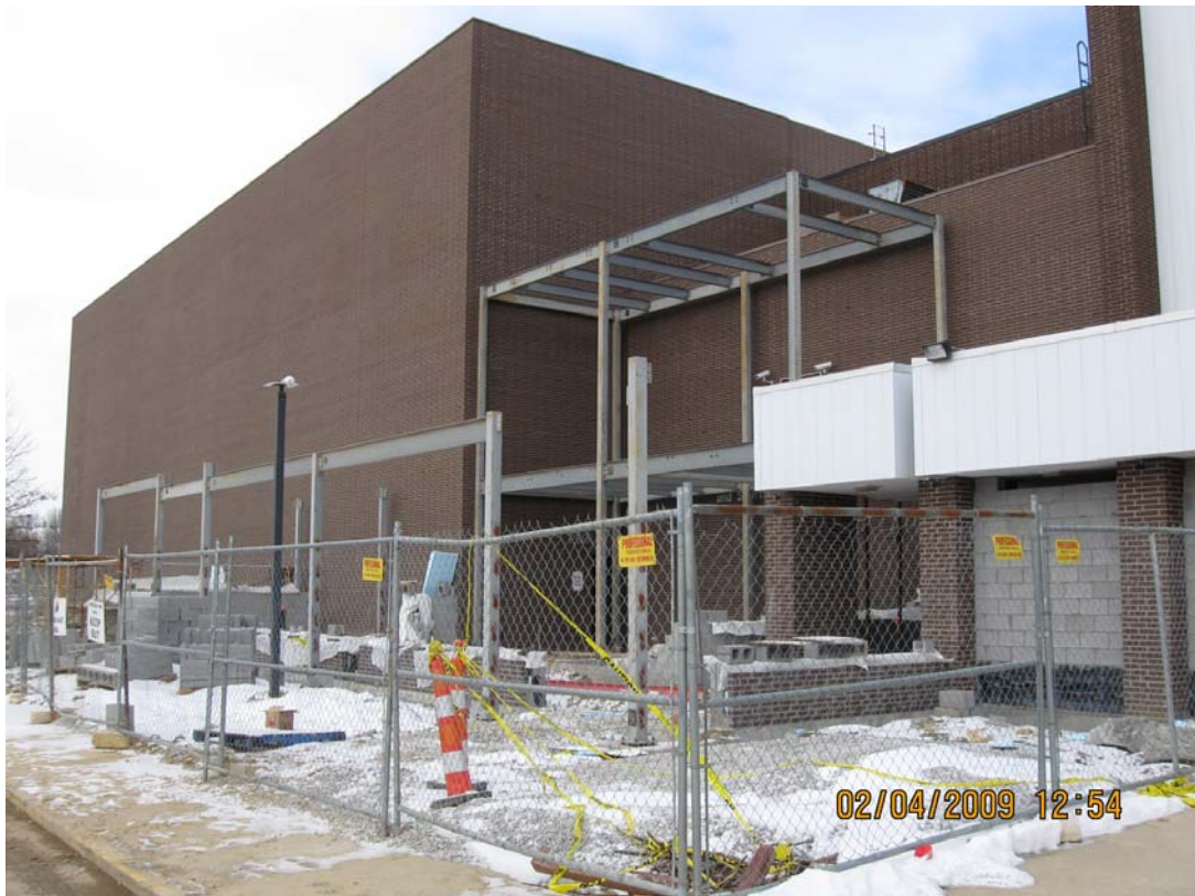
Erection of structural steel @ Vestibule / Mechanical Room Addition
