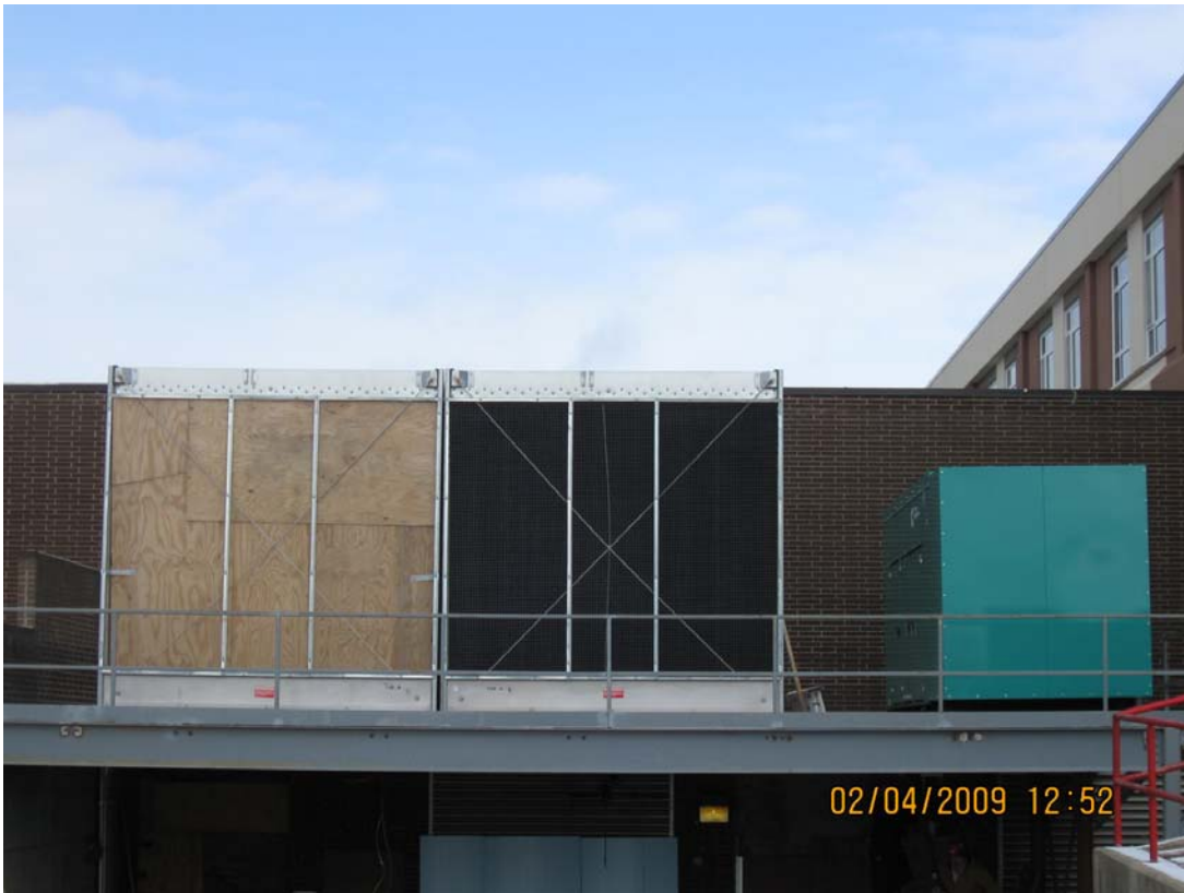
Setting of new Cooling Towers & Generator
