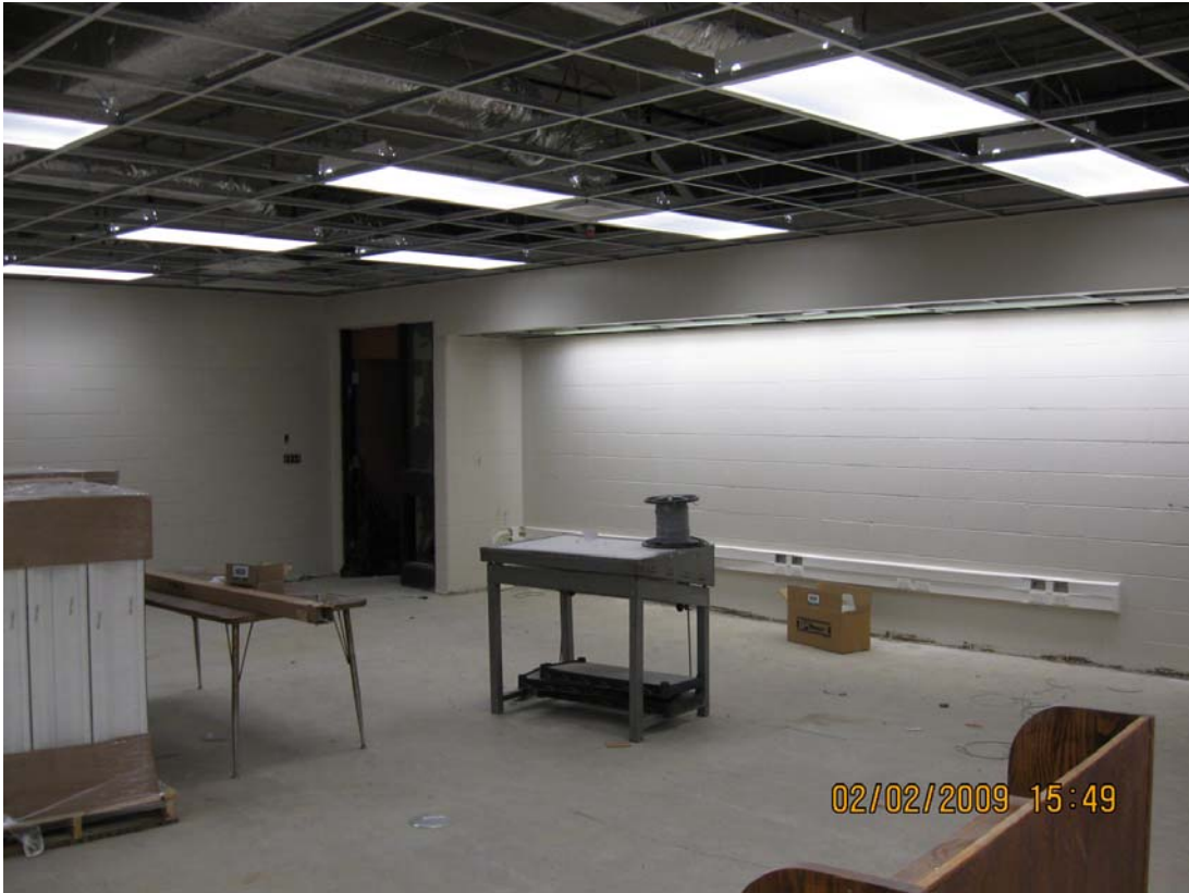
Renovation of 2 nd floor classroom
