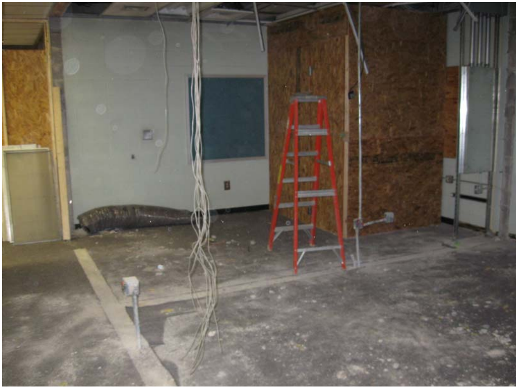
Demolition of Walls at Future MDF Room
