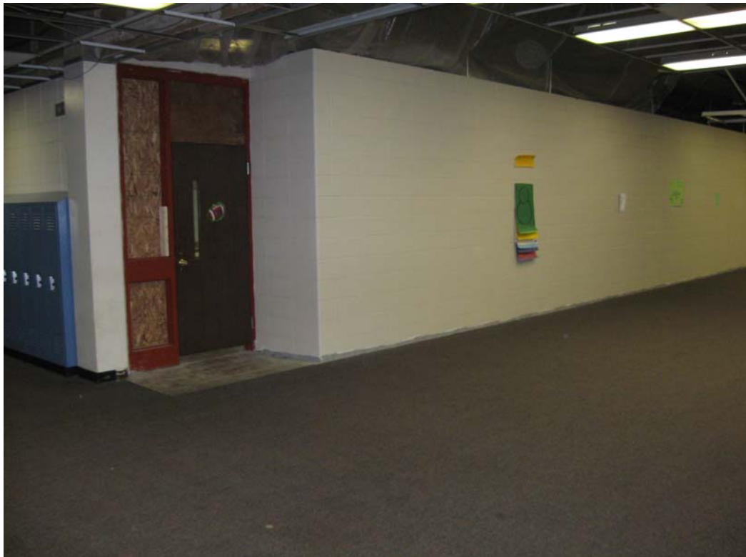
New Classrooms at Commons Area
