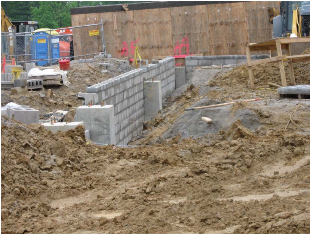
Building Foundations at Main Entrance Addition
