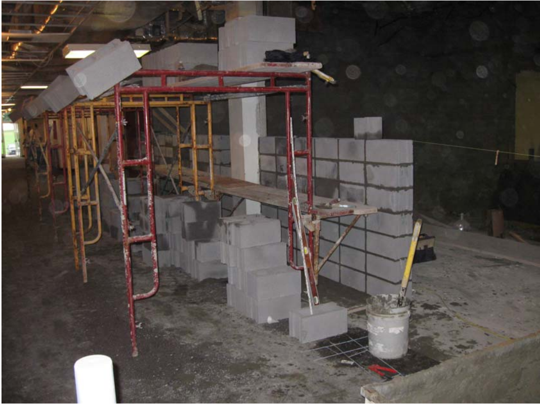
Erection of masonry at Unit C Science classroom
