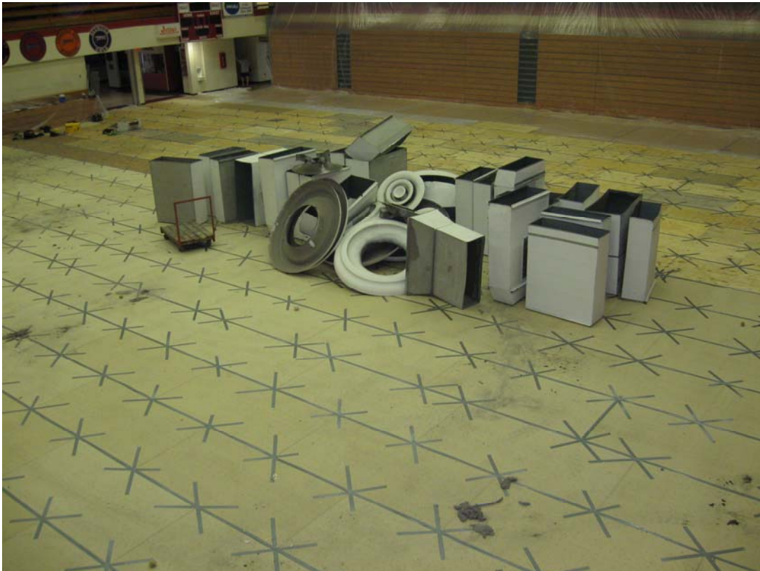
Demolition of HVAC at Gymnasium
