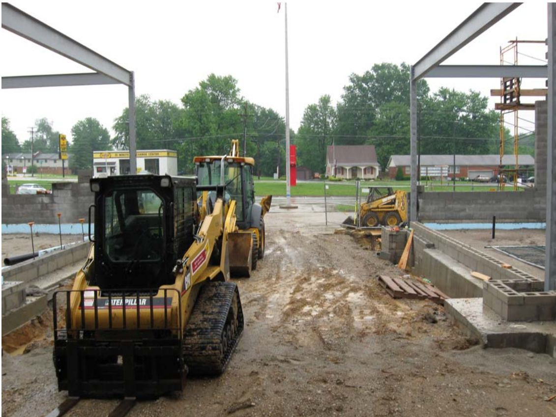
Removal of Main Entrance tunnel
