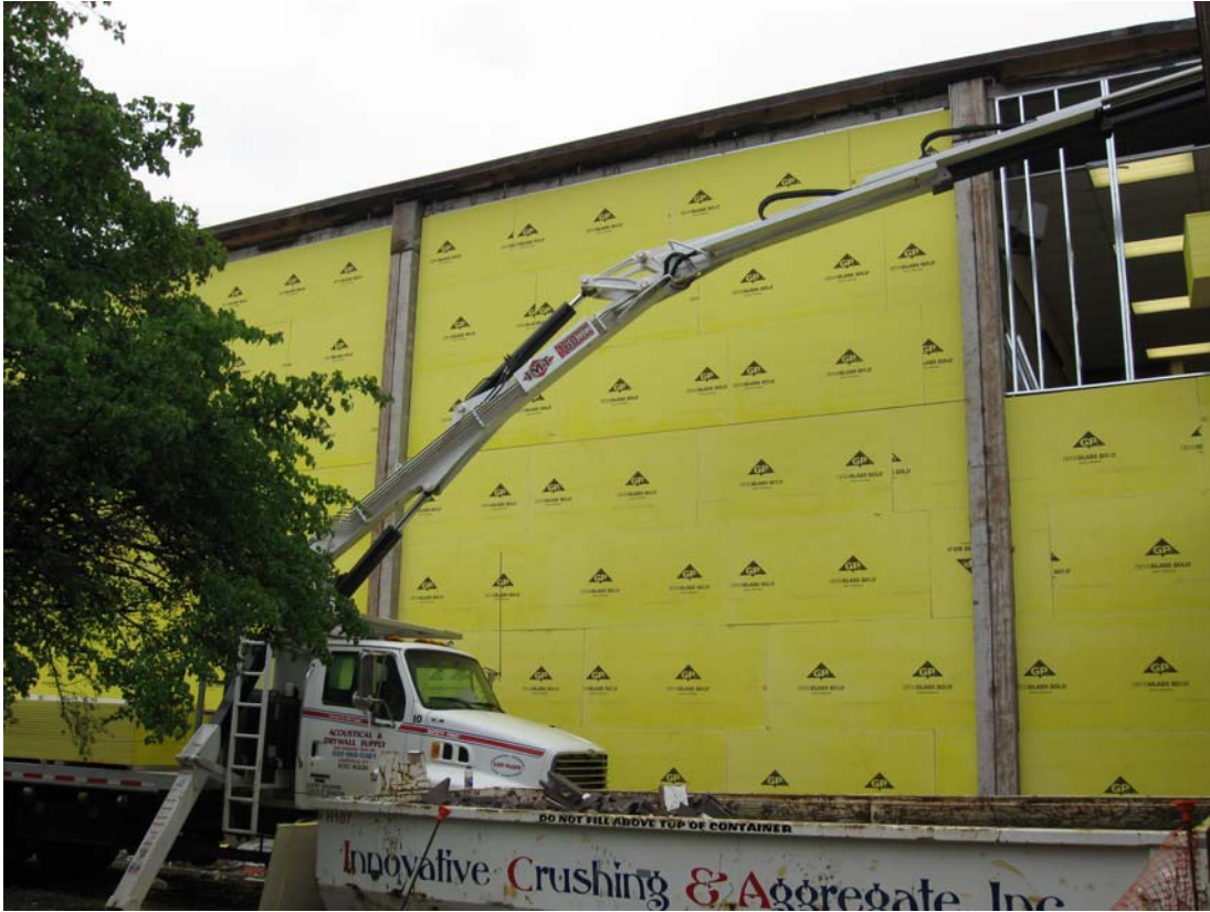
Erection of new skin along West elevation
