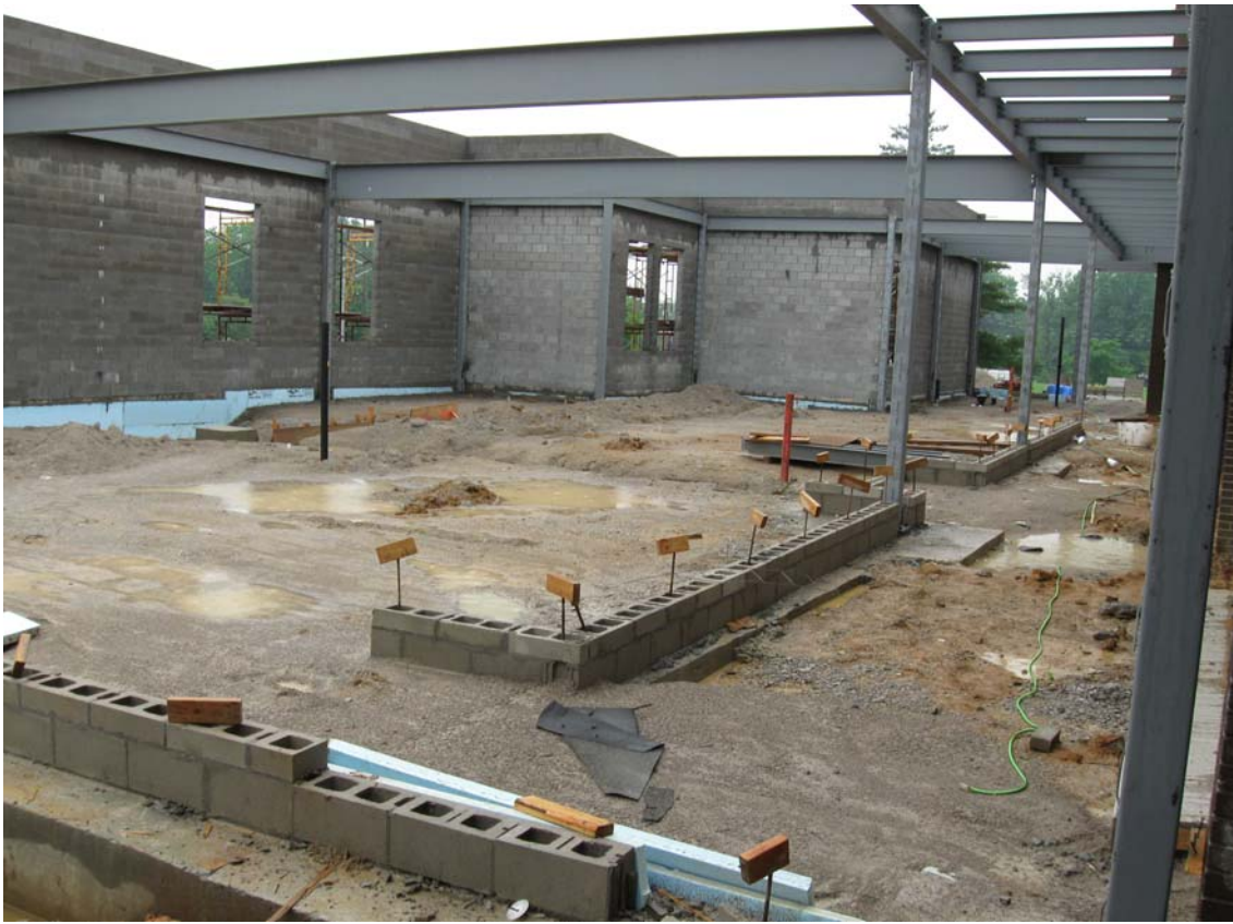
Erection of exterior walls and structural steel at Units A/B
