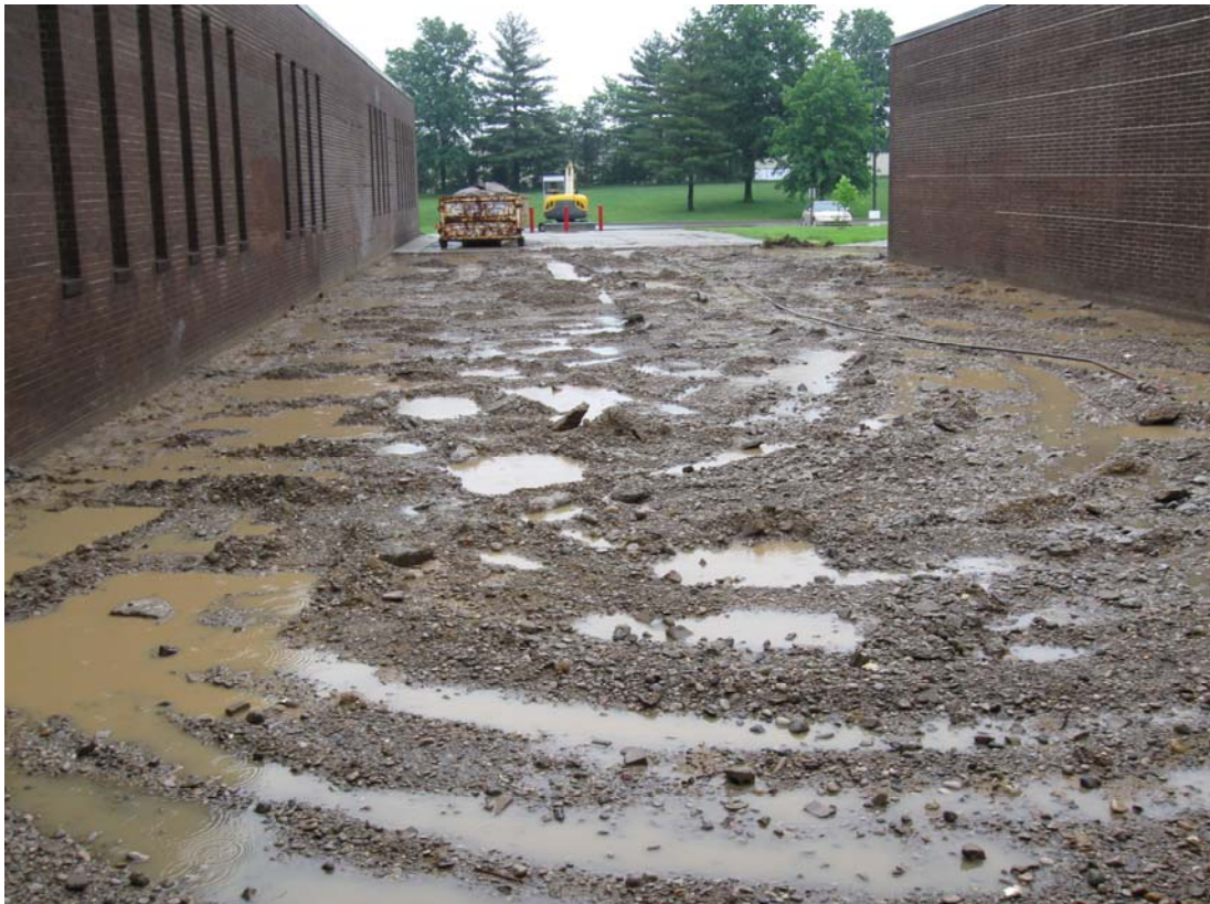
Demolition of Unit E entrance
