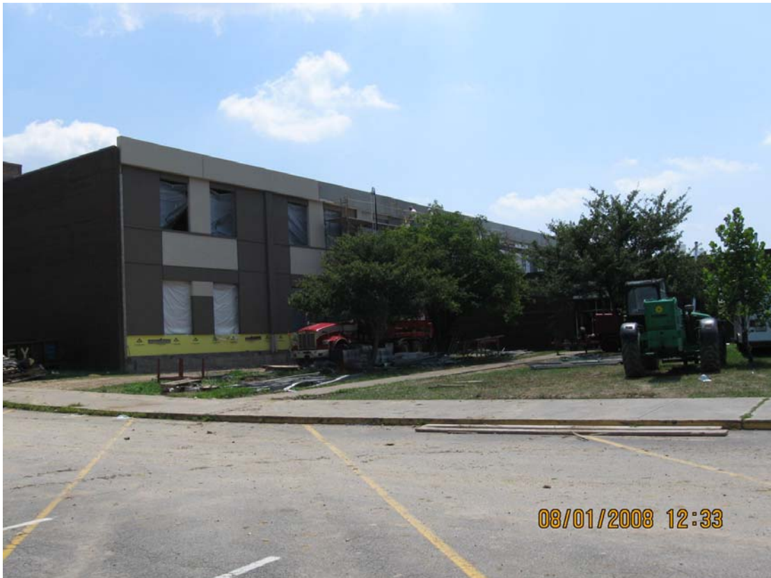
Installation of EIFS along West elevation
