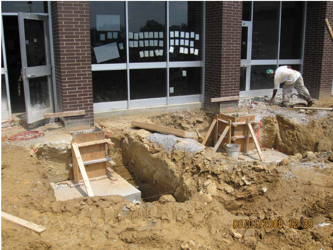
Building foundations at Cafeteria expansion
