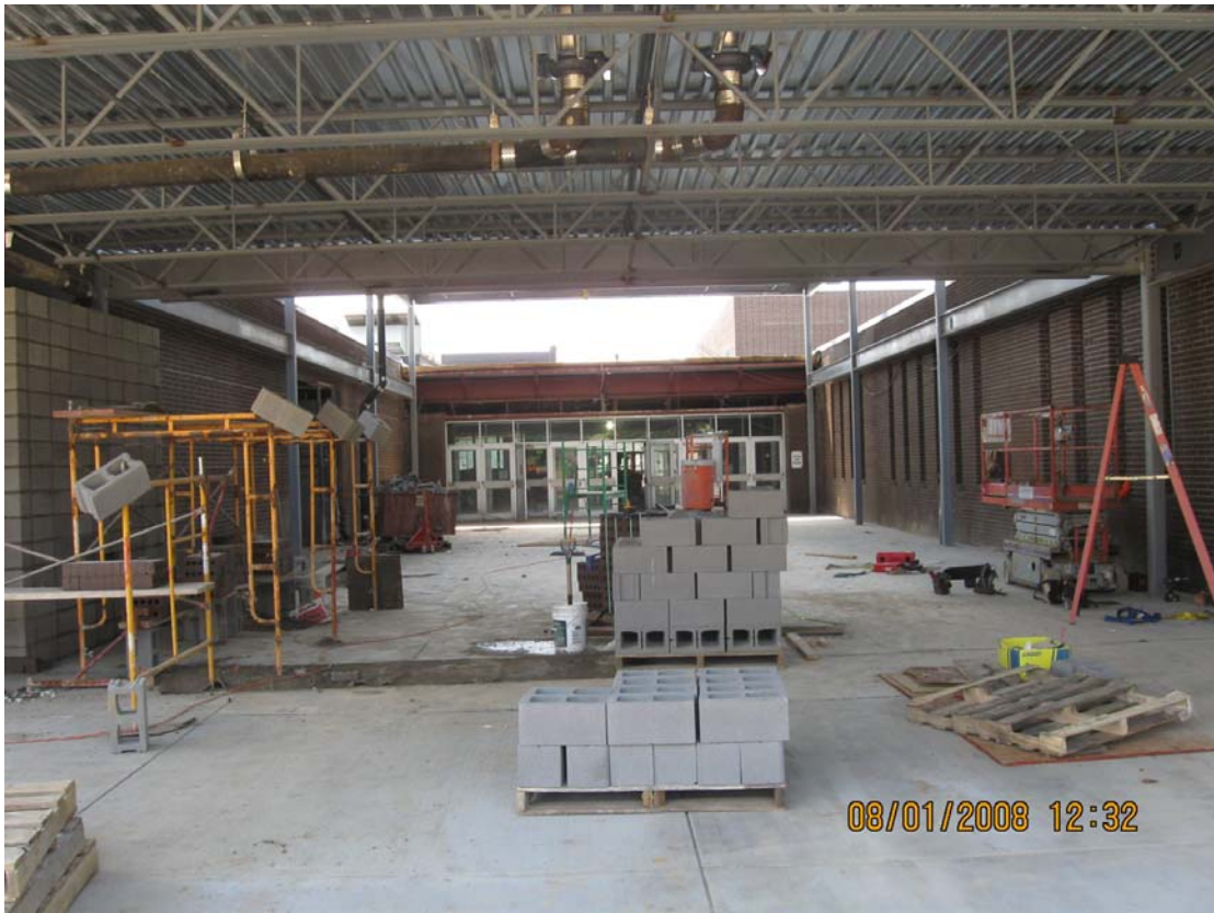
New Entrance to Unit E
