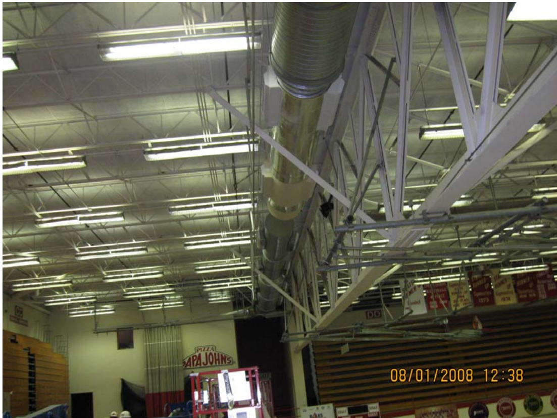
Erection of new ductwork within Main Gymnasium
