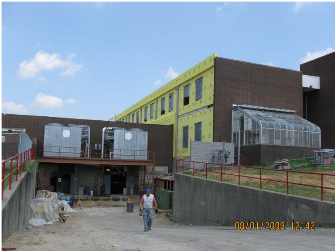
New exterior skin along West elevation
