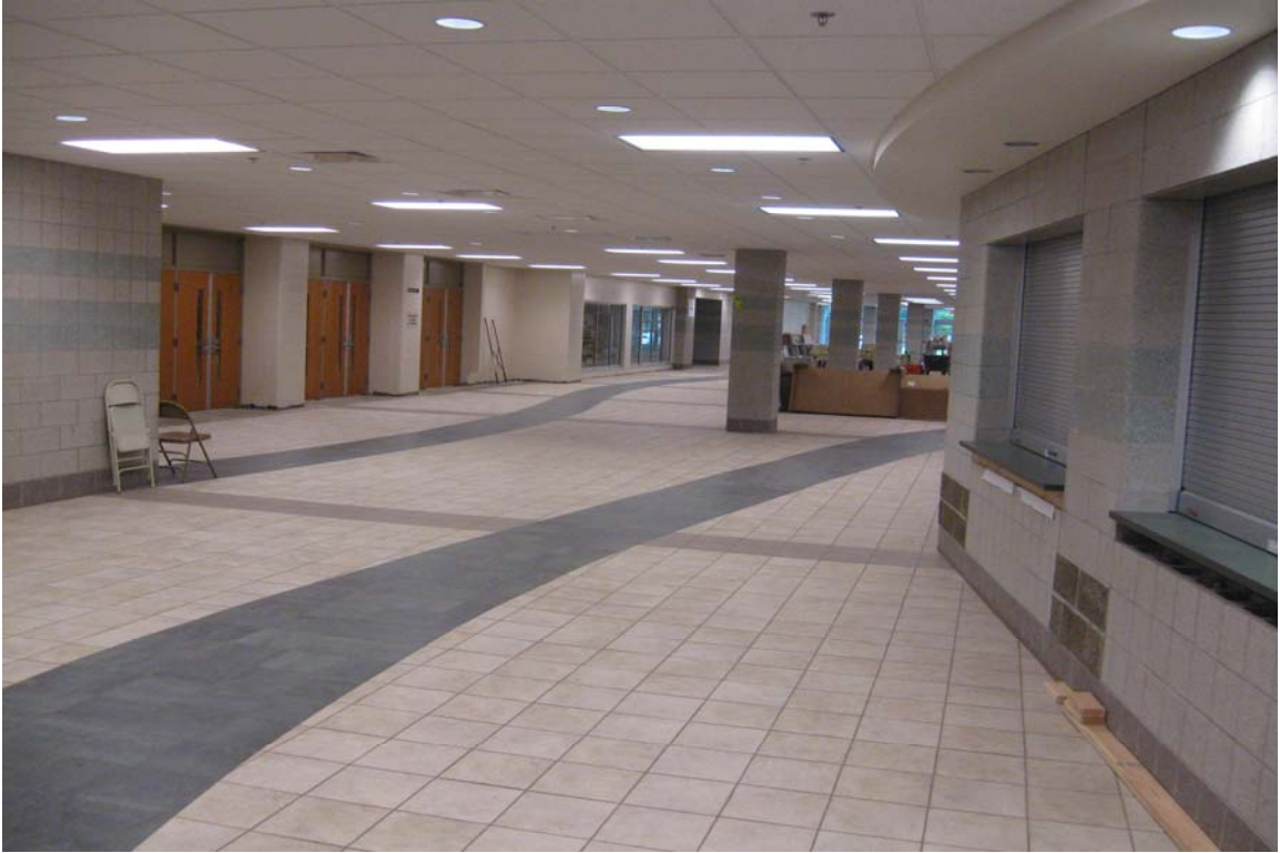
Ceramic Tile Flooring between Gyms
